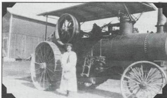
Steam Engine at Elmer Haier's Farm West Side of the Canal
