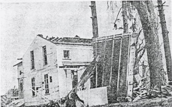
STORM DEPOSIT — A section heavily - damaged home along where two persons were killed of another building rests among the Meranda road, just east of by the tornado. the scalped trees in front of this the Mrs. Addie Zimpfer home,
