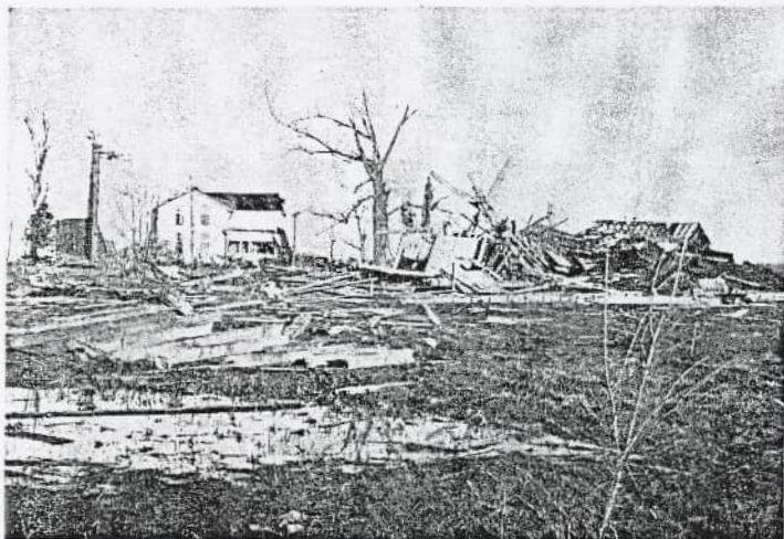
ALTHOUGH THE FARM home on a farm on Meranda road in the eastern portion of the county were torn asunder. The barn and other buildings located on the farm were completely destroyed. The distance the timbers from the structure were hurled. They can be seen in the foreground.
