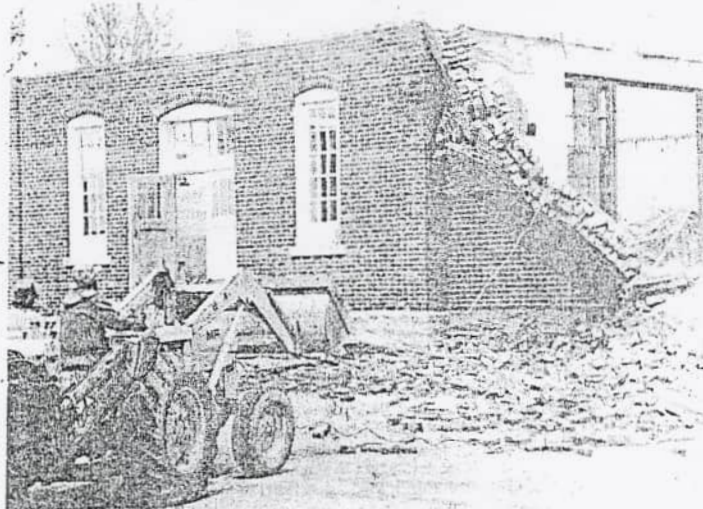
THE WALLS of St. Patrick School come tumbling down. The school held its first classes in the fall of 1908 and closed in the spring of 1954. Since that time, it has been used as
