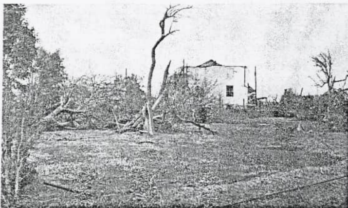
FRAMED BETWEEN what remains of trees is this farm house on the Meranda road from which the tornadic winds "gently" removed the roof, leaving the two lower floors standing. Damage to the house, however, was extensive.
