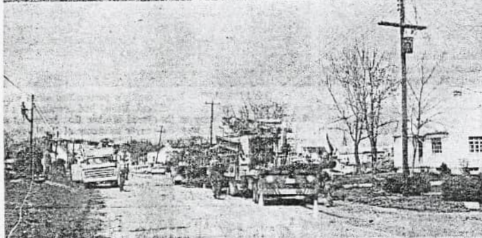
BUSINESS WRECKED — One of the establishments is shown in the top picture above. The lower photograph, taken in the same area, shows crews of the Dayton Power and Light Co. working along state route 66 to restore damaged service lines into the Fort Loramie community. The scene was one that could be found duplicated on many of the rural highways of the county for several days following the storm.
