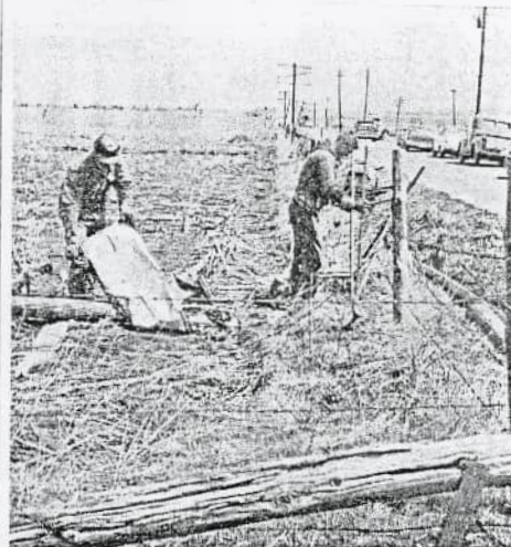
REPAIRS UNDERWAY — The areas laid waste by the Sunday night tornado. Telephone crewmen are shown preparing to reset a pole broken off on the Sidney - Freyburg road at the telephone and electric service to Meranda road.
