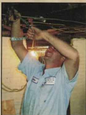
Installing New Heating System at the Parish Office
