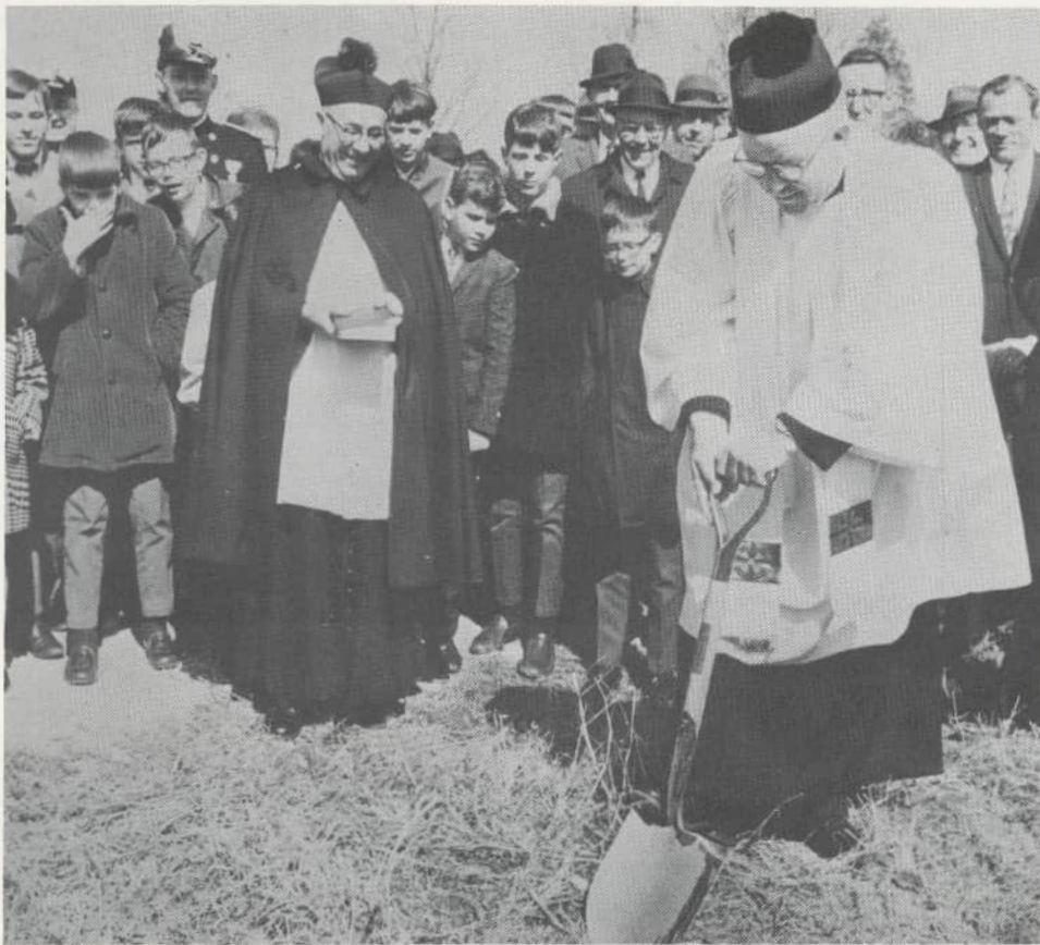
Groundbreaking of St. Michael's Hall
