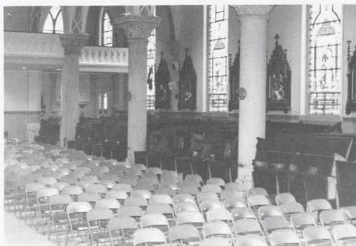
Church prepared for carpet laying-1988
