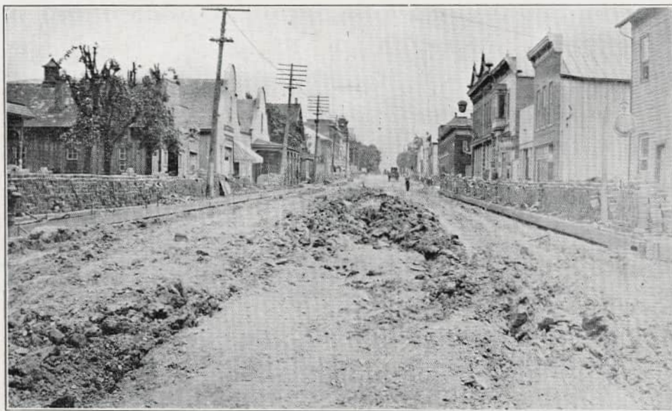
PAVING OF FOURTH STREET
