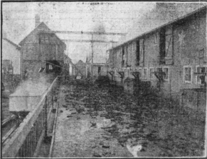
Cook house, food tank, cement trough and feeding floor.
