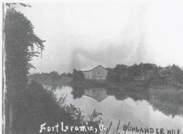
Bohlender Mill located at one time south of Ft. Loramie on Loy Road.
