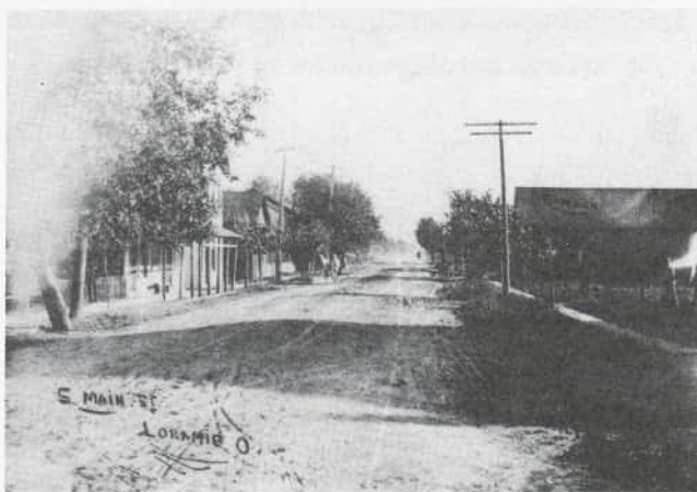
Early view of South Main Street looking south.
