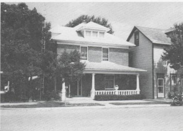
The Bernard Vogelsang, Vernacular style residence located 24 W. Main Street across the street from the Miami and Erie Canal Park. Ben Vogelsang operated the Vogelsang Cafe and his sons Elmer and Ralph carried on with the business. The building sits in the point of a triangle bounded by S.R. 66 the north by S.R. 705 and the west by the old Miami & Erie Canal. A bridge was over the canal in front of the building at one time.
