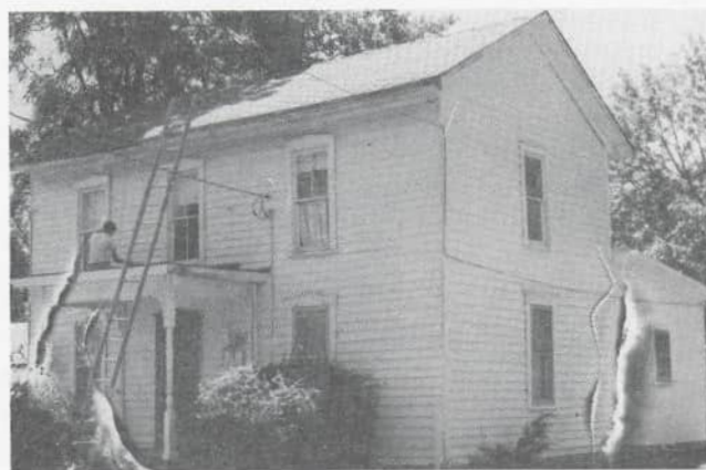
This Vernacular style home was built pre-1868. Located 48 S. Main St. This is the only house identified as a log house with walnut siding. The floor joist are hewn logs with flooring of two foot wide boards. It sits far back from the street, there was formerly a fence along the street and square limestone entrance columns and columns at corners of lot. The large front lot was utilized as a cow pasture. The old Miami & Erie Canal was within 50 feet of the back of the house. The home was occupied for a long time by the Burkhard Zimmerman family. Then was purchased by Albert Freytag. Herman and Elizabeth (Grothaus) Freytag lived there and their son Richard was born in the house during the depression. Ferd and Sylvia Freytag lived there with their children Julia and Philip from 1932-1937, then Albert Freytag sold it to Robert Freytag, his son. The home is now altered by a new owner with aluminum siding.
