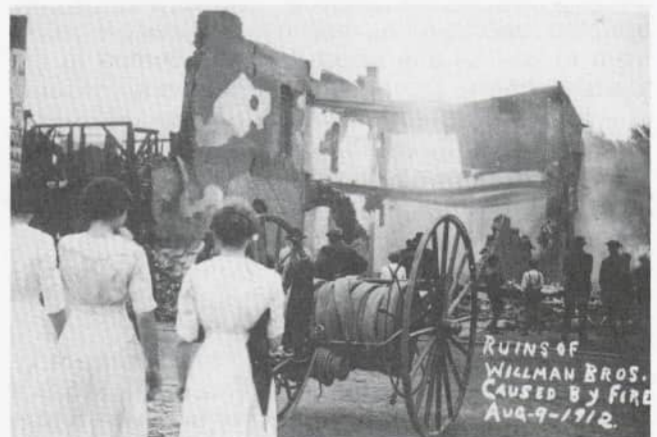
Fire, August 9, 1912 at Willman's Store and Home.
