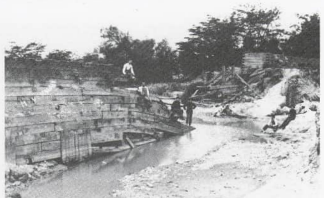
Broken Aqueduct. 1913 flood.
