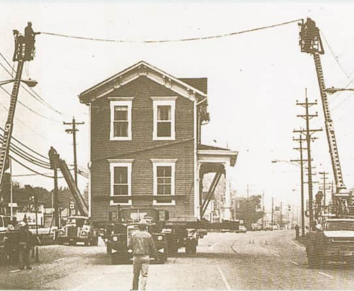
Immaculate Heart of Mary, Anderson Township (1944). To make room for the new church in 1978, the rectory was moved to a new location. Power wires had to be raised along Beechmont Avenue.
