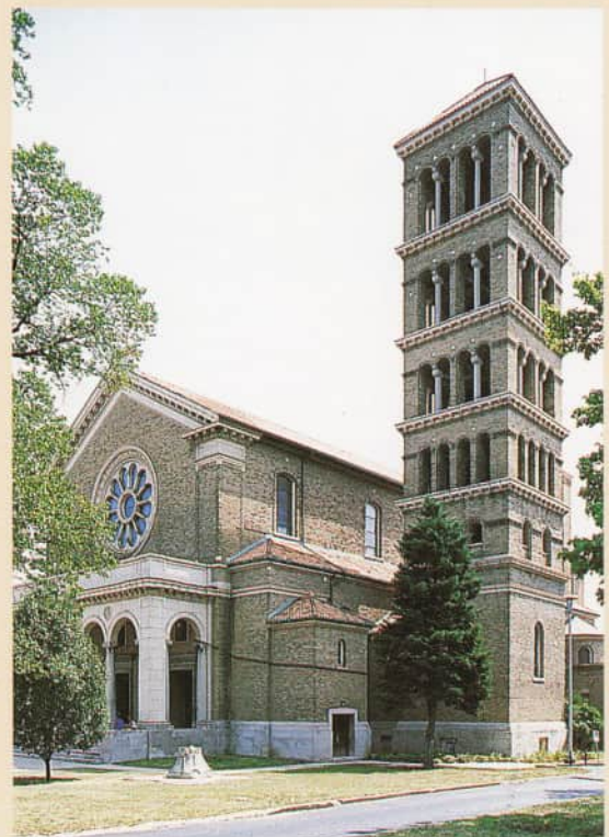
Church and campanile, St. Mark, Cincinnati (1905)
