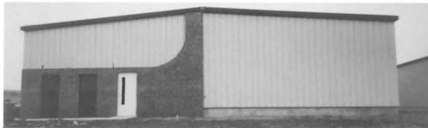
Present location of R & R Fabrications, Inc. still under construction. February, 1987.
