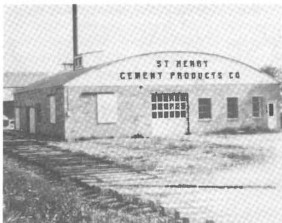
Laying new siding for Linus' factory – 1946.
