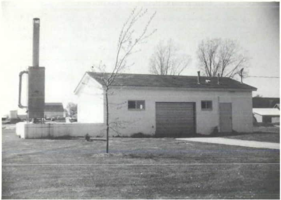
Water Treatment Building
