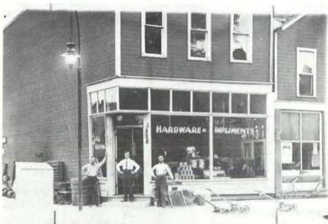
Hoyng Hardware. Frank Hoyng, Roman Hoyng, Joseph F. Hoyng. (White building at left was first gas station in Cold- water.)
