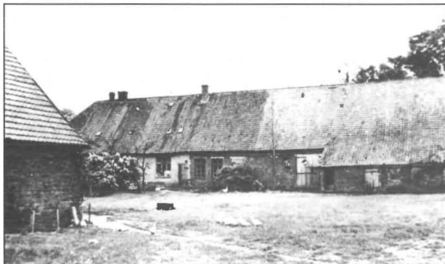
The Dicke house and barn at Heemsche.
