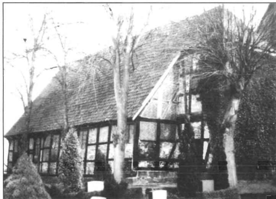
Front of the old church at Schinna.
