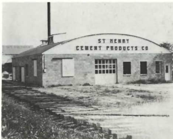
Laying new siding for Linus' factory. 1946.
