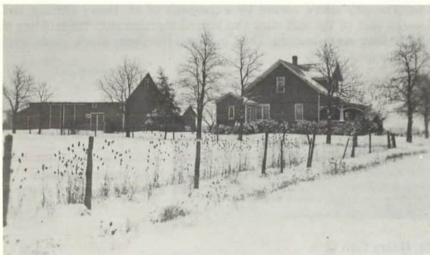
Gun Clubhouse in the north side of the barn behind Mrs. A. W. Bernard's residence, 321 East Kremer Hoying Road
