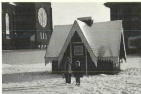
Santa Claus House, a project of Police Chief A. Bernard. 1971
